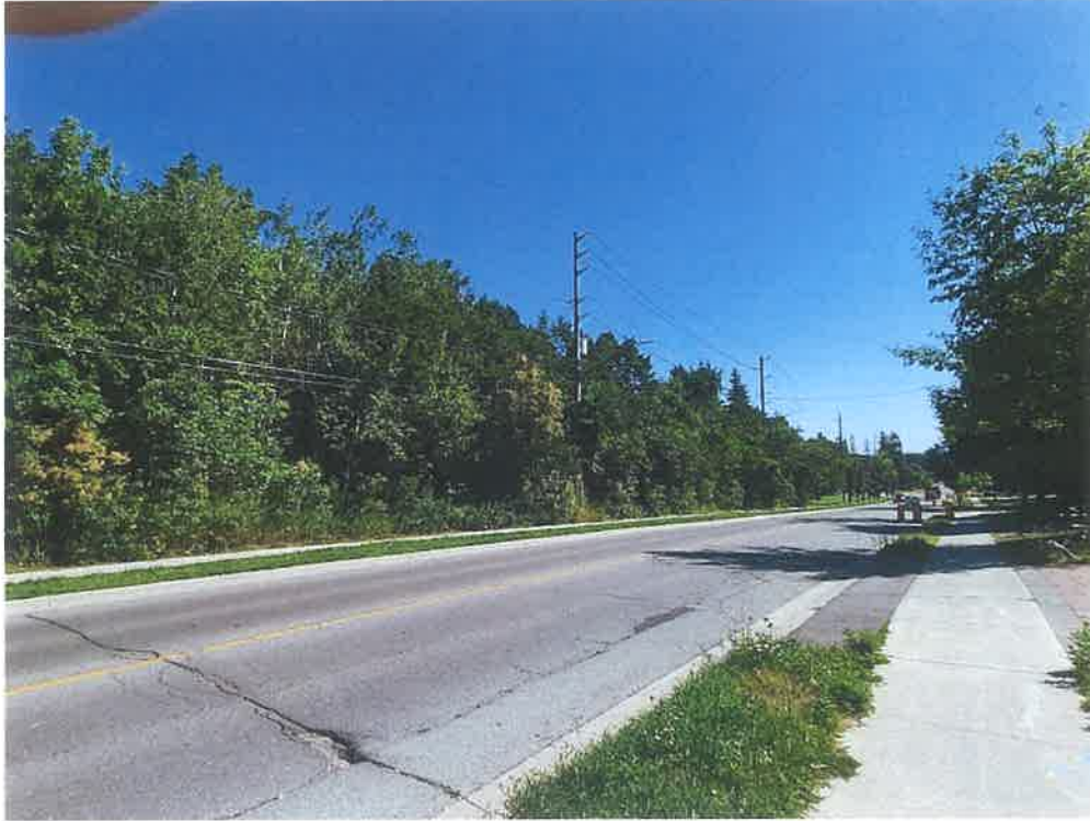
A general view of wooded south side of the subject site (looking northeast)
