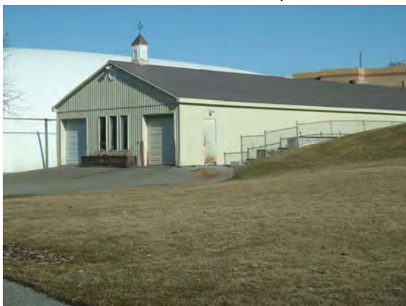
Plate 5: Maintenance buildings associated with the club house.
