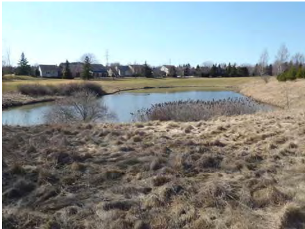
Plate 7: Storm water management pond/water trap within Section C, south of the golf course.
