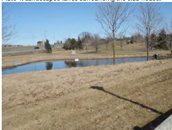
Plate 6: Storm water management pond/water trap within Section C, north of the golf course.
