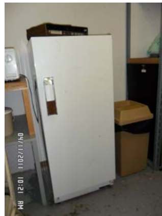
Photo 4: Old refrigerator possibly containing ODSs in sprinkler room in clubhouse
