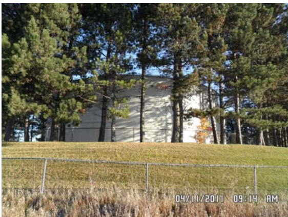
Photo 17: Pump reservoir, facing south
