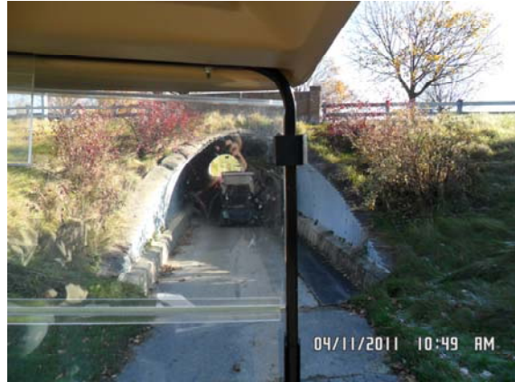
Photo 14: Golf course tunnel under Eagle Street
