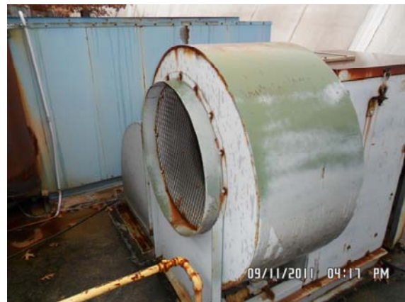
Photo 10: Blowers associated with indoor tennis dome
