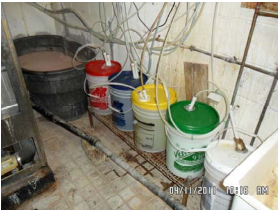
Photo 3: Chemicals in laundry room in clubhouse
