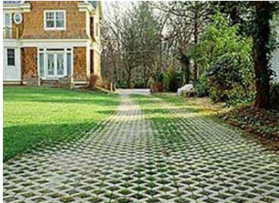
Porous pavement in residential driveway
