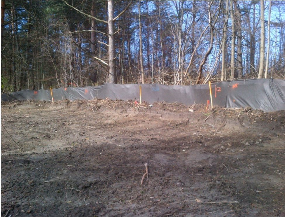
Photograph 3: Excavated Remediation at Area A.
