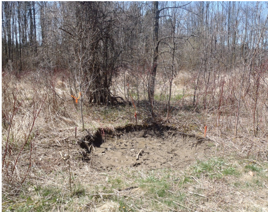
Photograph 8: Excavated Remediation at Area F.
