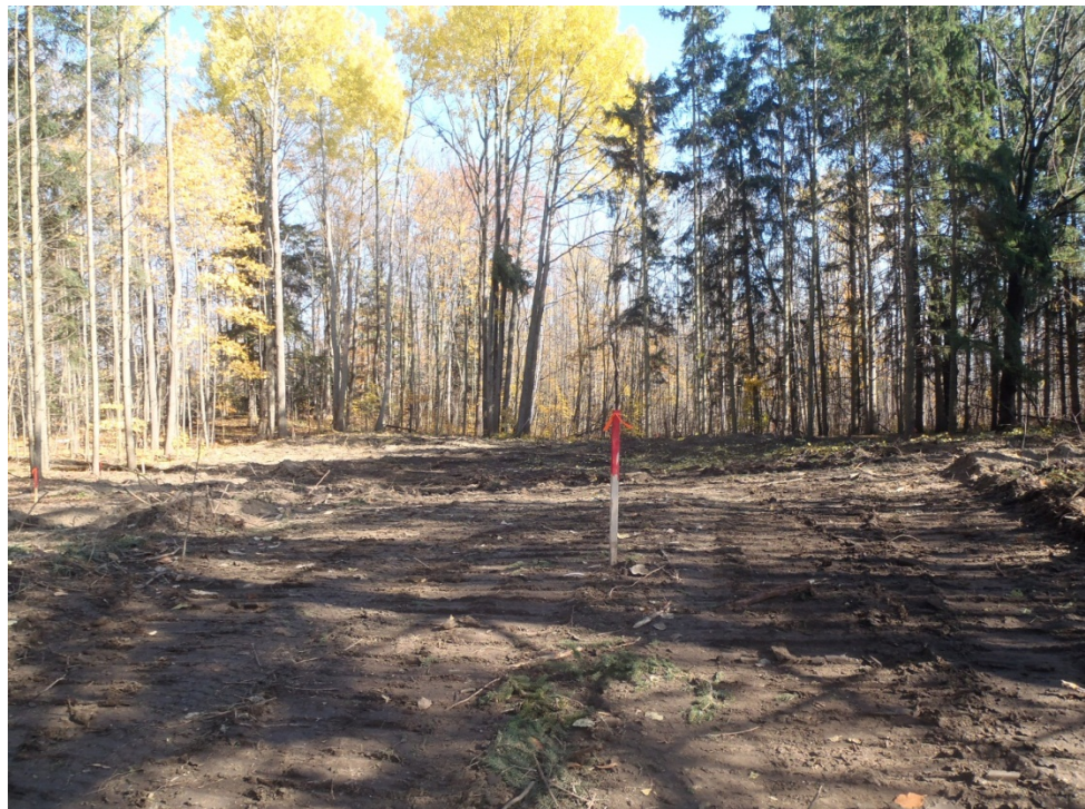
Photograph 6: Excavated Remediation at Area D.
