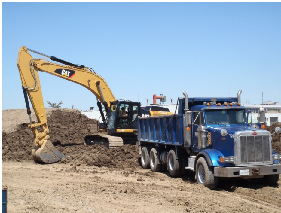
Photograph 9: Replacement topsoil being loaded at source site – 1030 McNicoll Avenue.
