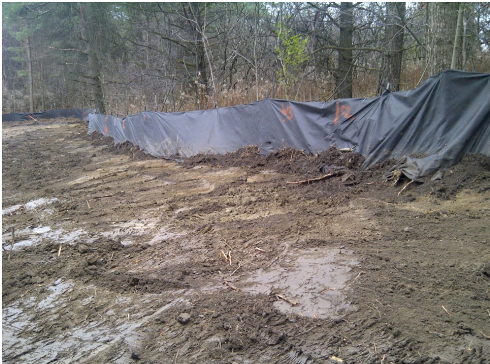
Photograph 4: Excavated remediation at Area B.
