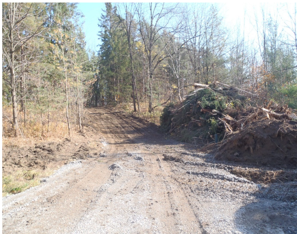
Photograph 10: Dense vegetation evident beyond access road at Area D.
