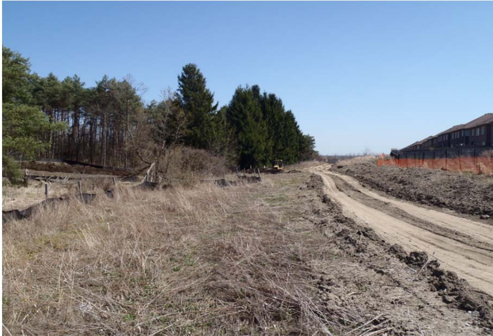
Photograph 1: Access road to Areas A, B and E.
