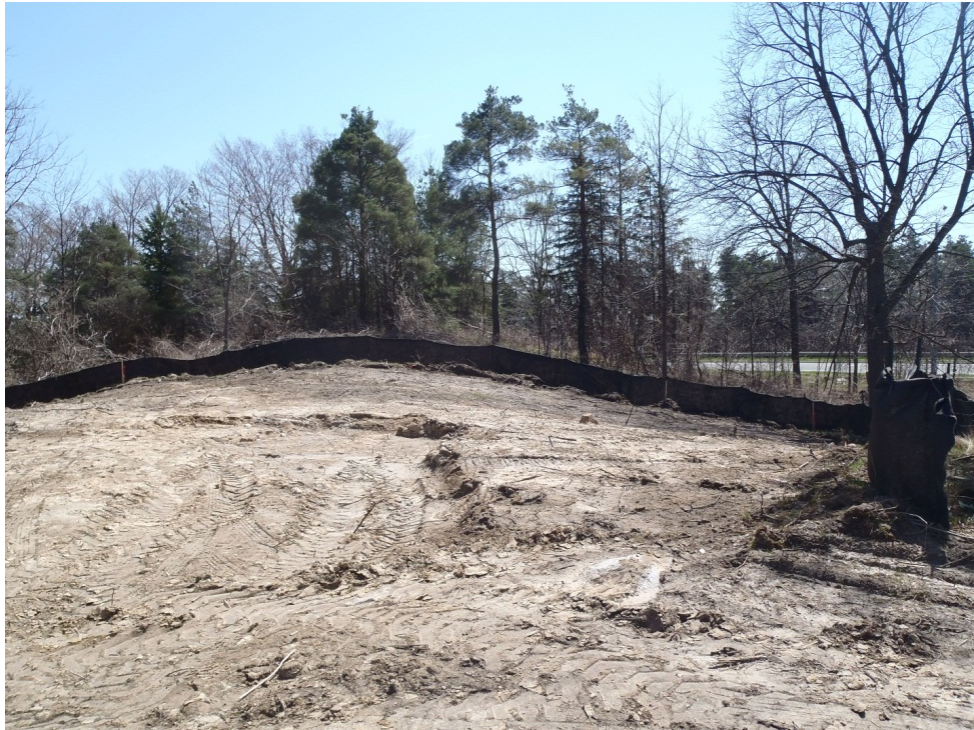
Photograph 5: Excavated Remediation at Area C.
