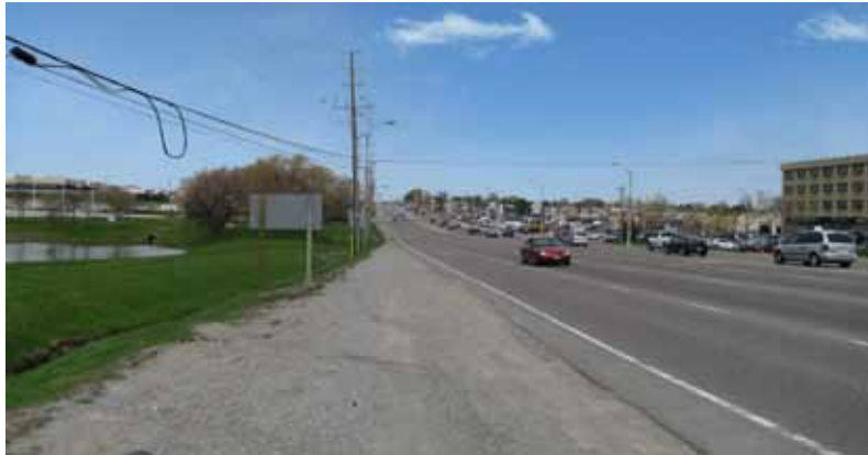
3. Yonge Street Looking North of Davis Drive
