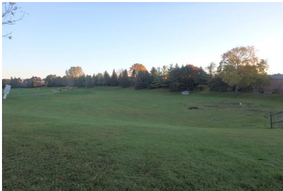
Dry Stormwater Pond (Newmarket), AECOM
