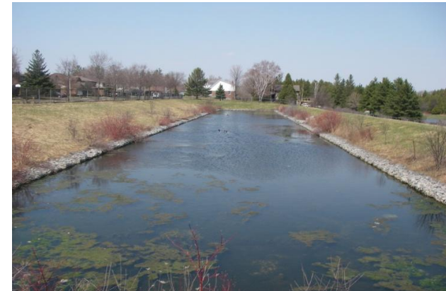
Wet Stormwater Pond (Guelph), AECOM
