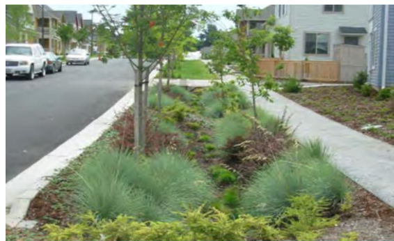
Bioretention Swale – "Grey to Green Road Retrofits", Credit Valley Conservation
