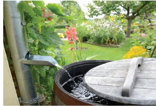
Residential Rain barrel, Credit Valley Conservation
