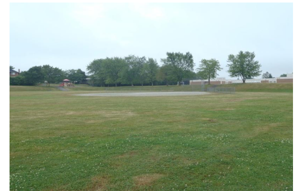
Dry Stormwater Pond (Guelph), AECOM
