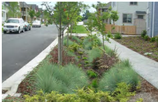
Bioretention Swale – “Grey to Green Road Retrofits”, Credit Valley Conservation
