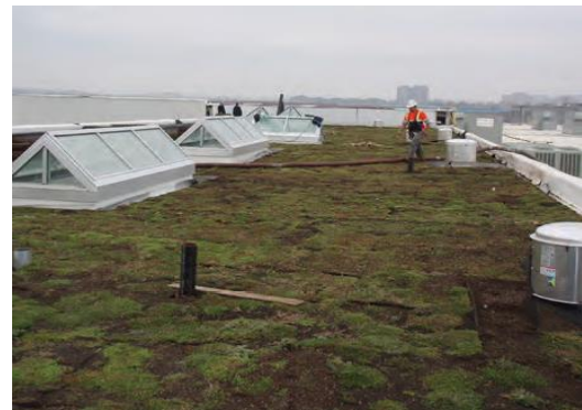
Green Roof, Credit Valley Conservation
