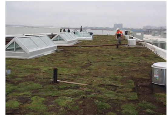
Green Roof, Credit Valley Conservation
