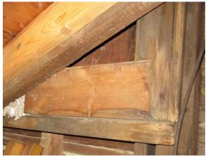
Blocked up finished window to framed house in roof crawl space of brick extension (ERA).
