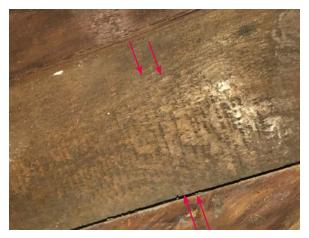
Bandsaw marks in wood on rafter in timber frame building (ERA).
