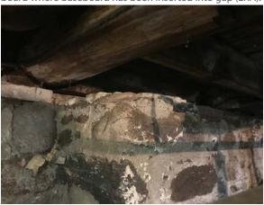
Base of hearth in cellar. Note framing around opening for hearth to extend into ground floor (ERA).
