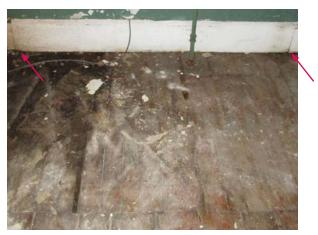
Flooring infill repair where hearth has been removed on ground floor of brick extension. Note visible lines in baseboard where baseboard has been inserted into gap (ERA).
