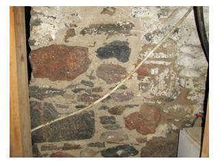
Cellar walls. Note lime rich mortar from later addition next to softer and darker mortar from earlier constraction(ERA).
