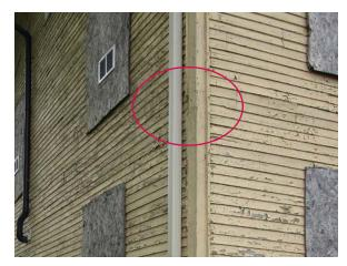
Patching of original trim on East elevation where the porch was removed (ERA).
