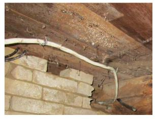
Top of arched support in cellar. Note how it stops short of the floor structure (ERA).
