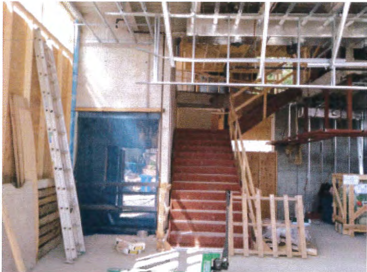
Elevator installation has commenced, stair at reception installed
