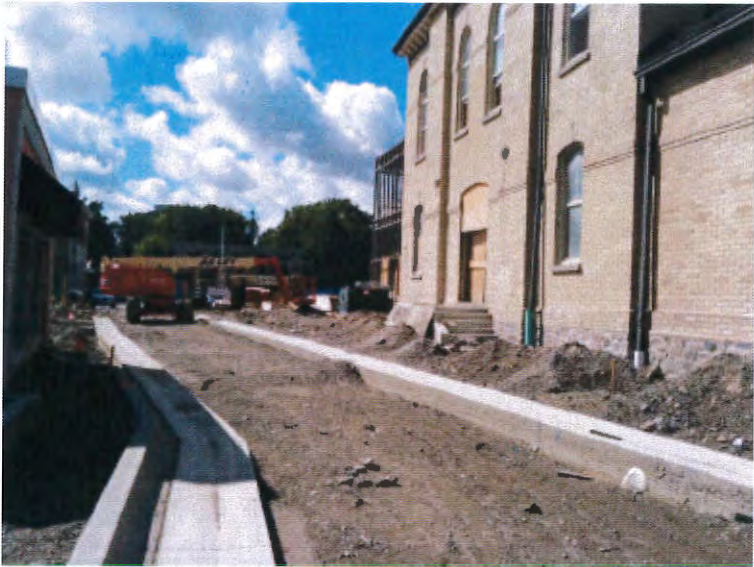
East Lane hard landscaping has commenced
