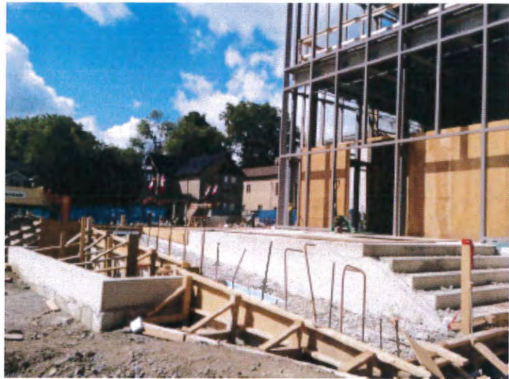
Podium at south entrance is underway
