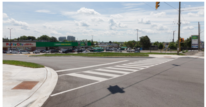
New traffic signals at the entrance to Canadian Tire and the Food Basics Plaza improve access and traffic flow.
