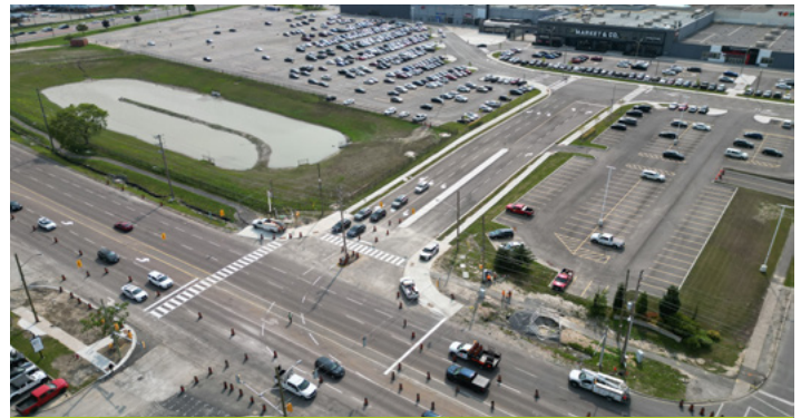
Relocated traffic signals at Upper Canada Mall for better alignment and to accommodate future residential development.
