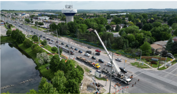
Through a partnership with NT Power, 68 hydro poles were installed along the two-kilometre corridor.
