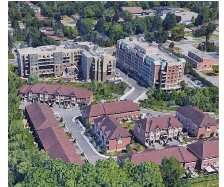
Townhouses and mid-rise apartment buildings at Doak Lane
