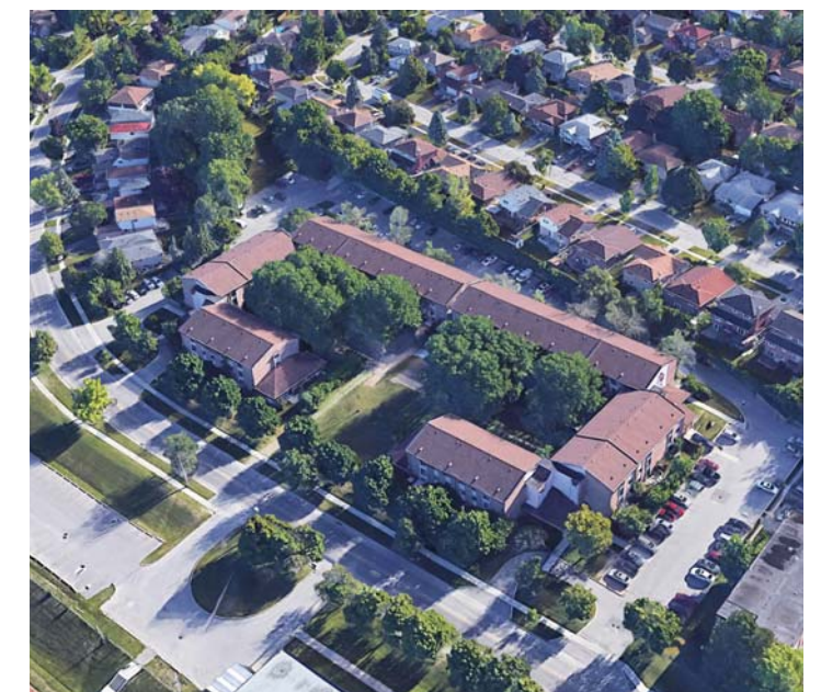
Low-rise apartment complex at Huron Heights Drive
